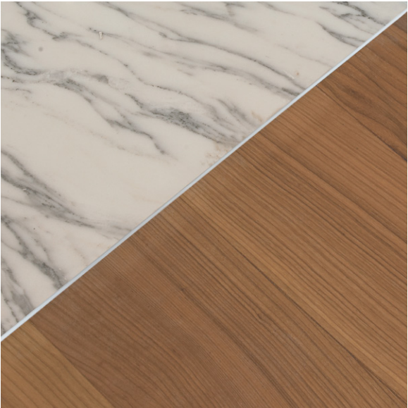
Threshold Joint - Stainless Steel
